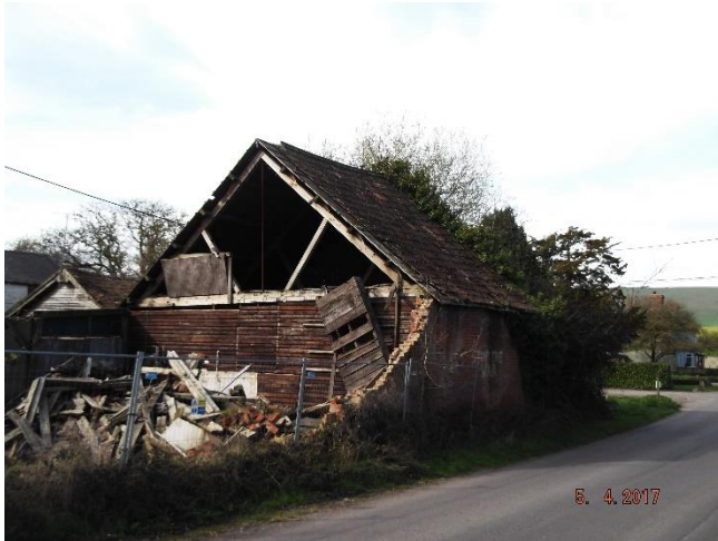
View of existing roadside building
