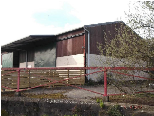
View of building to west of site from Canal
