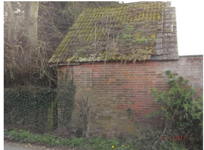
View of existing roadside building
